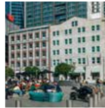
2017 Australis Nathan Buildings 12 refurbishment is completed.
