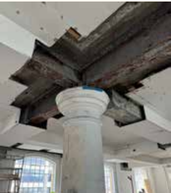
Above ‘Sawtoothing’ floorboards around the columns where reinforcing was needed helped conceal the interventions.
