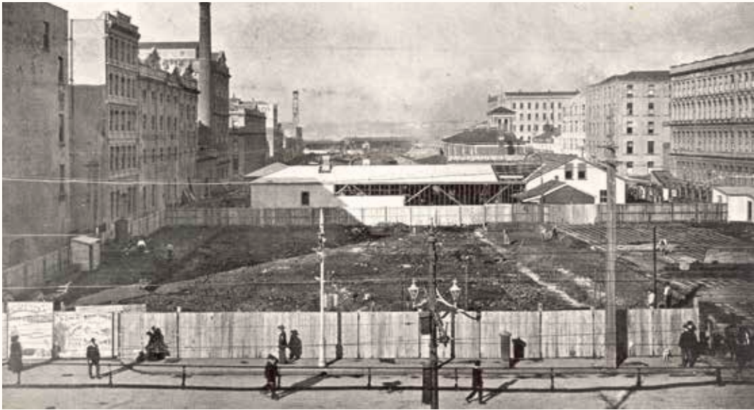
Left A 1909 view of preliminary construction work for the new Chief Post Office on the site of the former Queen Street Railway Station, looking east. Photo from the Auckland Libraries Heritage Collections 323161
